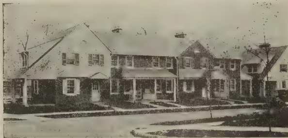
FIG. 12—BUCKMAN VILLAGE, CHESTER, PA.— ROW OF TYPICAL HOUSES G. EDWIN BRUMBAUGH, SIMON & BASSETT, ARCHITECTS
